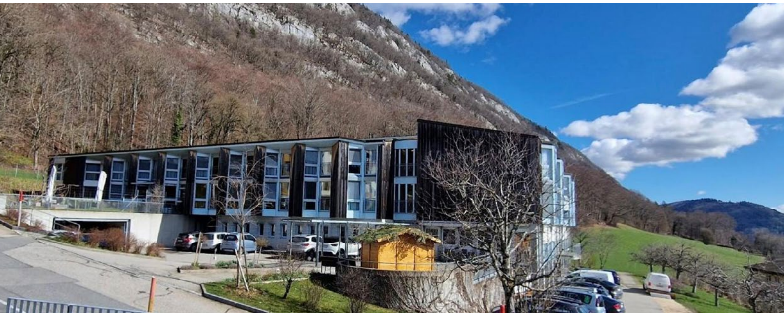
Residential Care Facility Les Roches, Orvins, Switzerland
